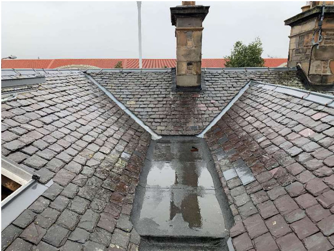
View from roof of built up felt valley gutter as well as degradation to flashings.
