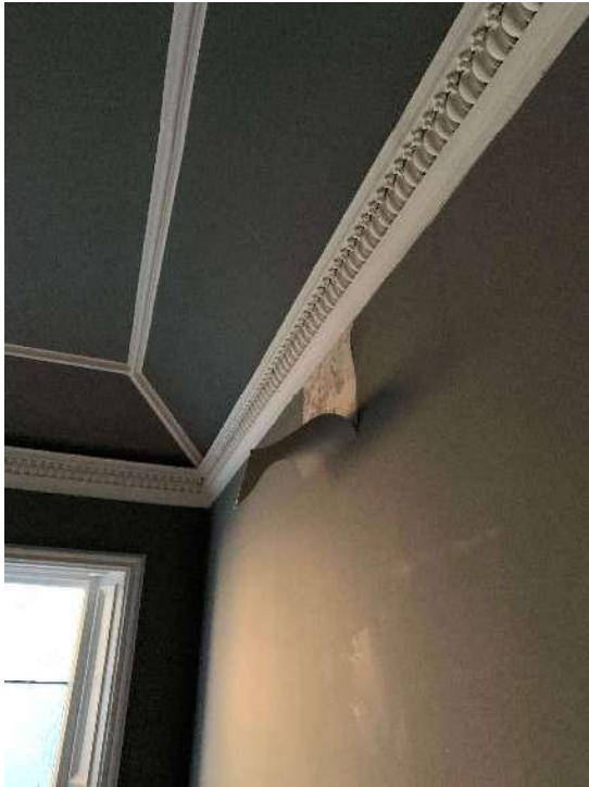
View from upper landing showing the extent of water ingress
