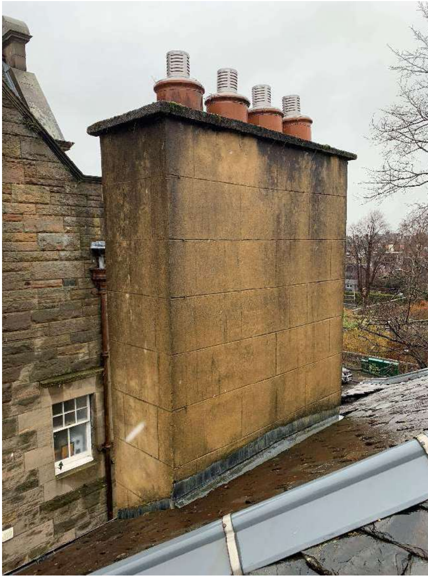
View from roof showing poorly constructed chimney on west elevation.
